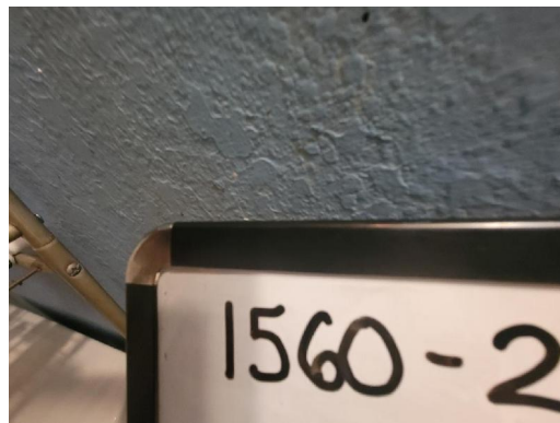
1560-2 Joint Compound/Drywall Typical Interior Walls/Ceilings
